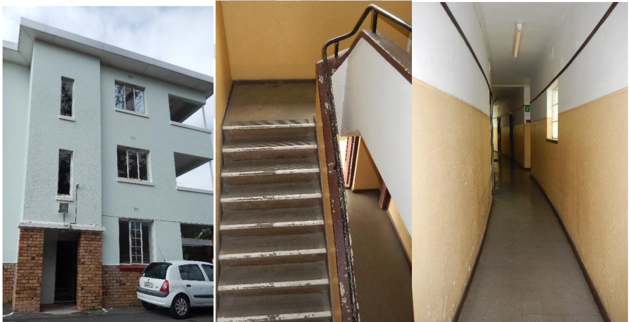
FIGURE 3: Narrow entrances, staircases and corridors
