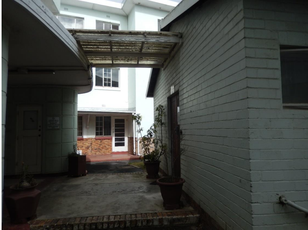
FIGURE 2: Additions to the main structure
