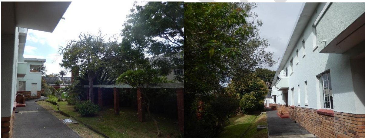
FIGURE 1 B: Back façade of Werverdiend (22 Rouwkoop Road)
